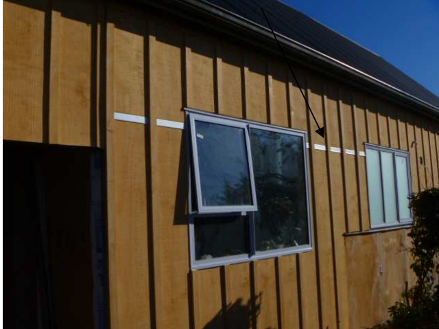
New cladding to barn, note horizontal flashing
