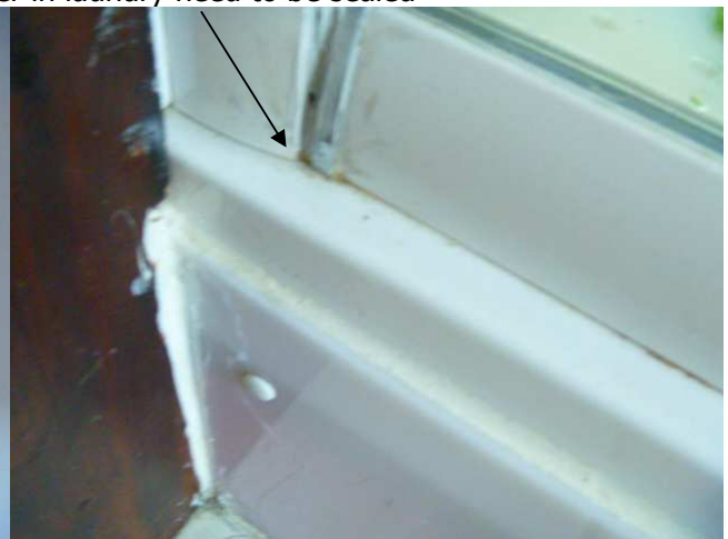
Leaks from corners of shower in laundry need to be sealed
