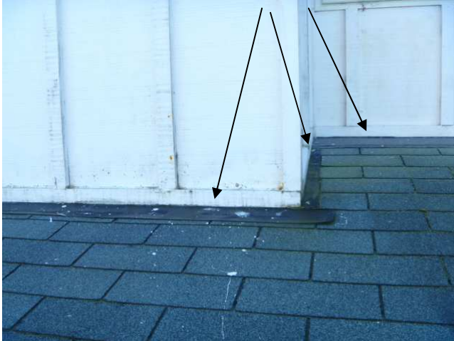
Cladding finished hard down onto roof flashing will rot in time
