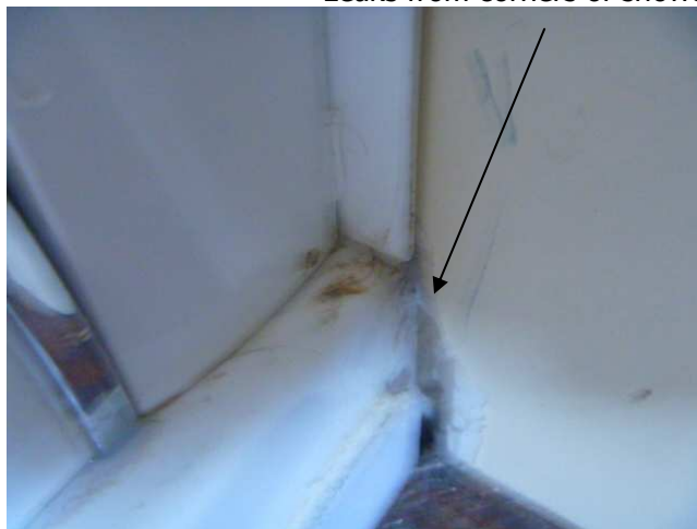
Leaks from corners of shower in laundry need to be sealed
