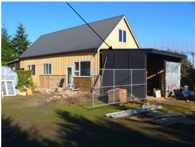
Lean-to at end of barn
